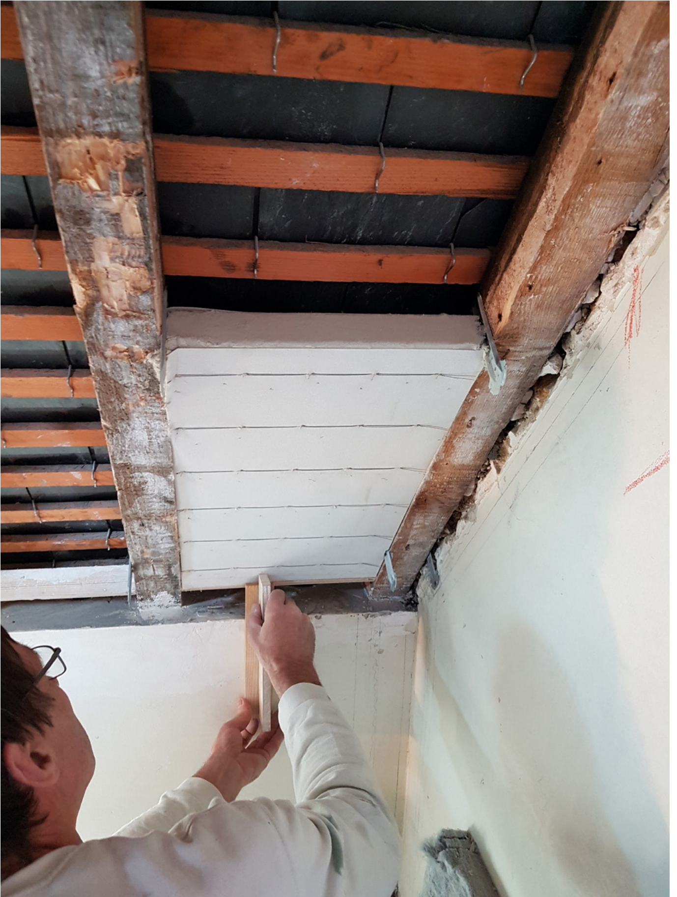
CALOSTAT® Sandwich F as insulation between the rafter combines high insulating performance and fire protection in a single material.
