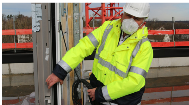
Franz Ebert of FKN points out the slim design – just 90 mm of the actual facade Foto: Evonik/F. Gmach
