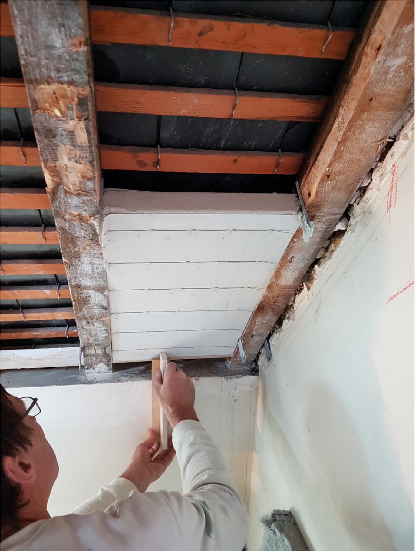
*CALOSTAT® Sandwich F as insulation between the rafter combines high insulating performance and fire protection in a single material.*
