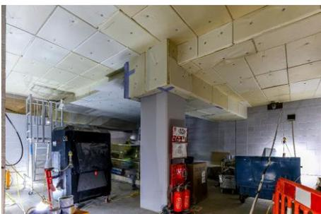
Thin, non-combustible insulation for the basement ceiling at One Nine Elms Street in London.
